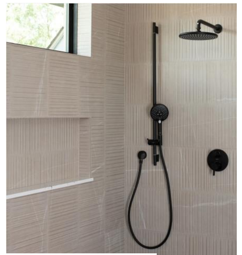
INSTALLATION IMAGE: SHOWER WALL TILE (T-3)
